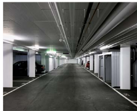
Parking souterrain (200 places)
